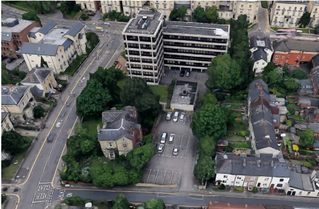
Aerial view looking north towards Kings Road
