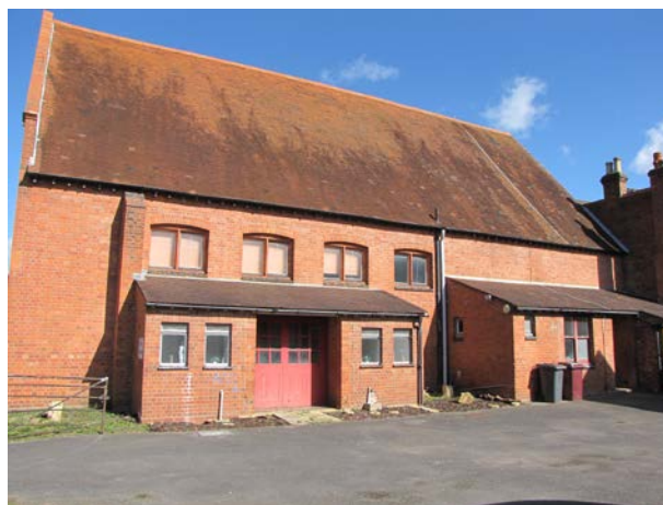
Rear elevation of church
