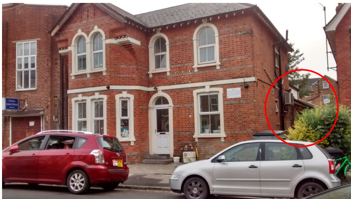
Site in current view from Waylen Street. Unauthorised extension is just visible in the red circle. Front boundary wall is missing.
